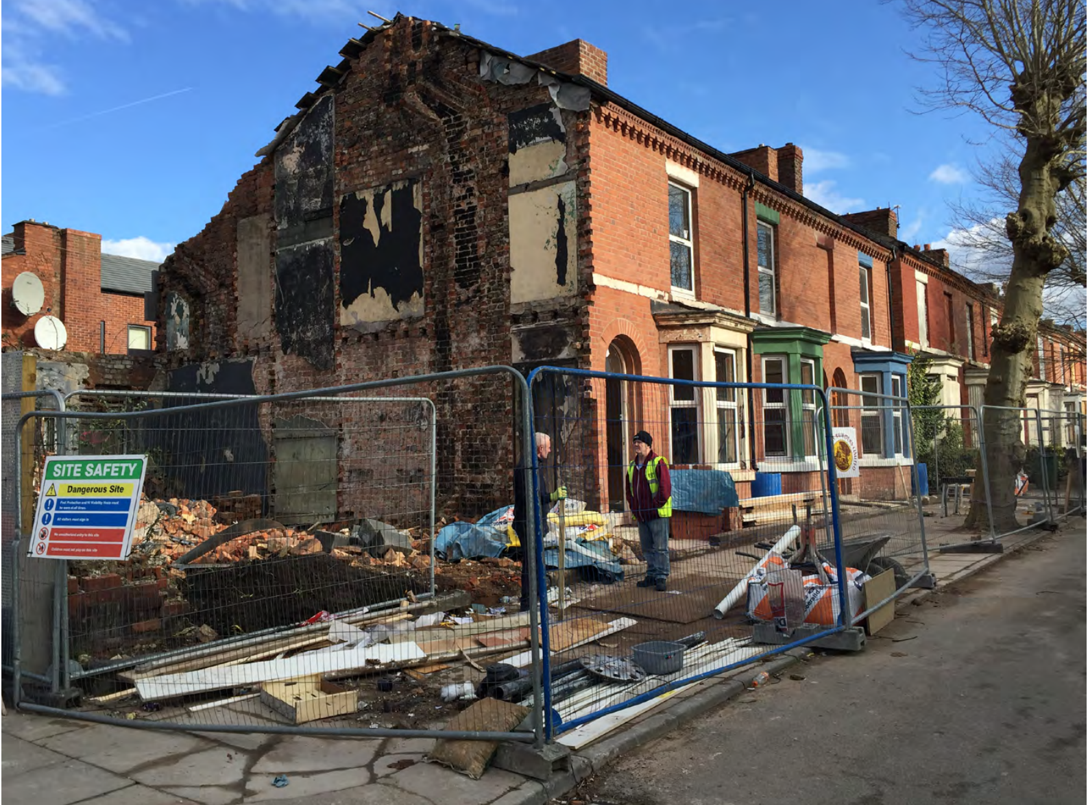
Construction works. Photo © Eutopian
